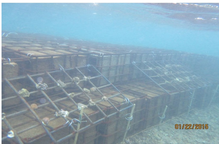
Figure 20. A hybrid CR4 structure installed in Grenada to reduce wave energy. Photo credit: TNC.
